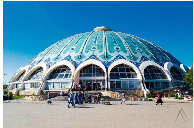
Chorsu dome bazar in Tashkent
